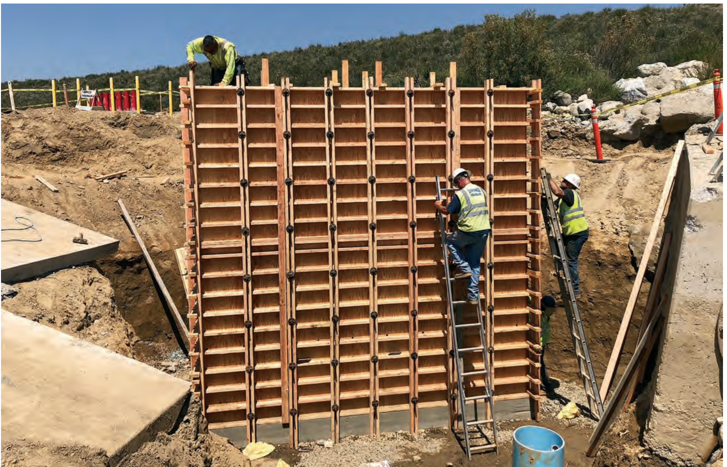
Construction underway at San Sevaine Basin.
