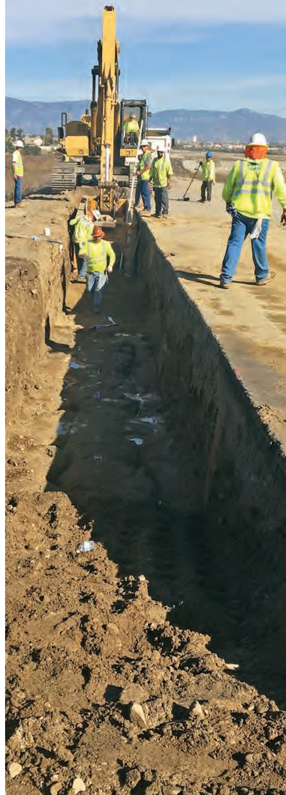
Trenching for pipelines to connect recharge basins.
